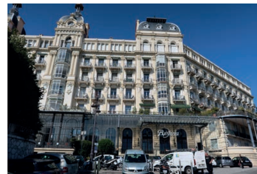
Excelsior Regina Palace (1897) (MH) S.M Basini,
